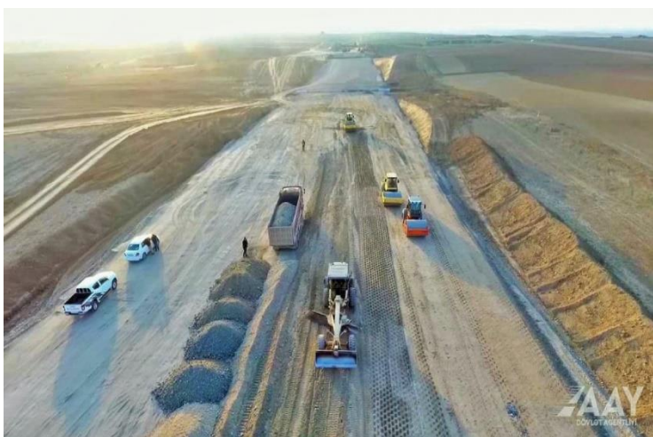
Pic 3. The construction of the Ahmadbayli-Fuzuli-Shusha highway.
